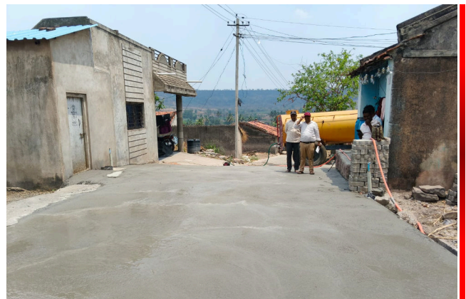
Road constructed by women's group
